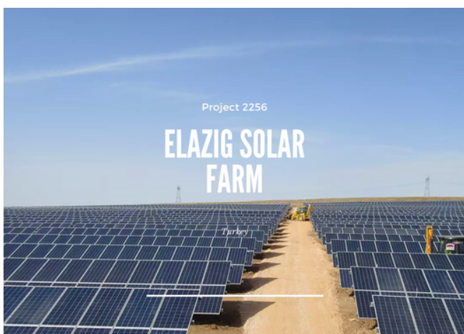
Project 2256: Elazig Solar Farm in Turkey
