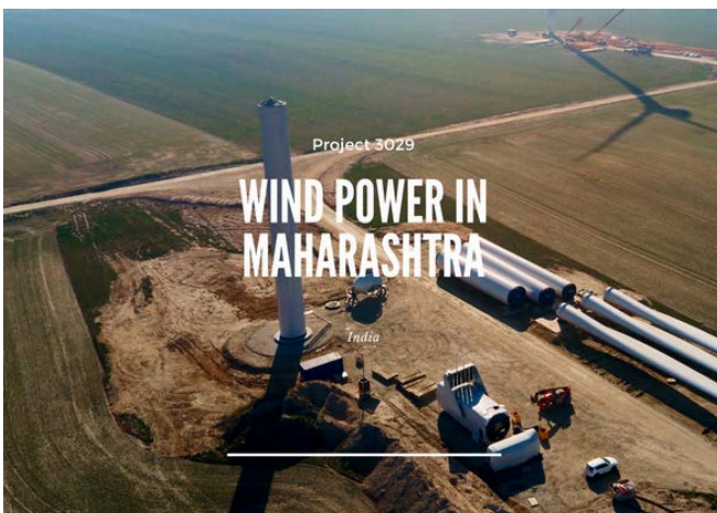
Project 3029: Wind Power in Maharashtra
